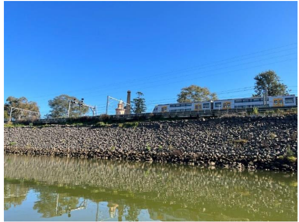
Left: opposite bank – severe erosion common. Right: opposite bank – rock armour along rail corridor.
